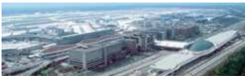
Frankfurt Int. Airport | Germany
